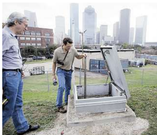
Kevin Shanley, left, and Guy Hagstette prepare to climb into the hatch on top of the reservoir's artificial hill near downtown.
